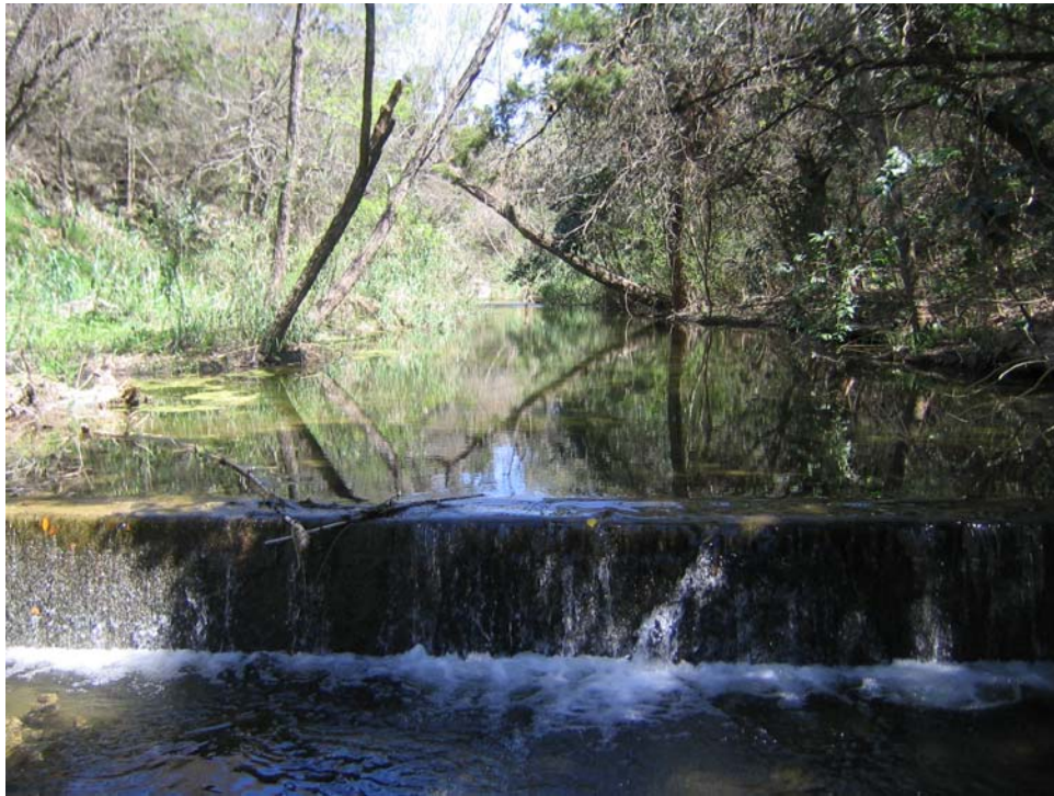
Figure 46: Native Stone Steps and Concrete Spillway Dams
