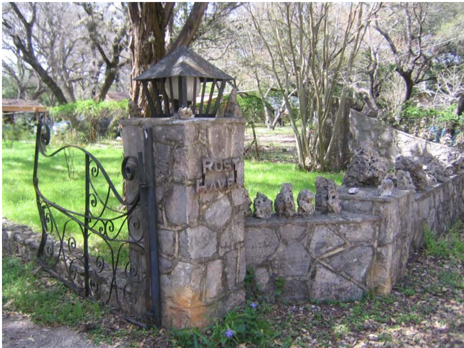
Figure 54: Stone Walls and Wrought Iron Gates
