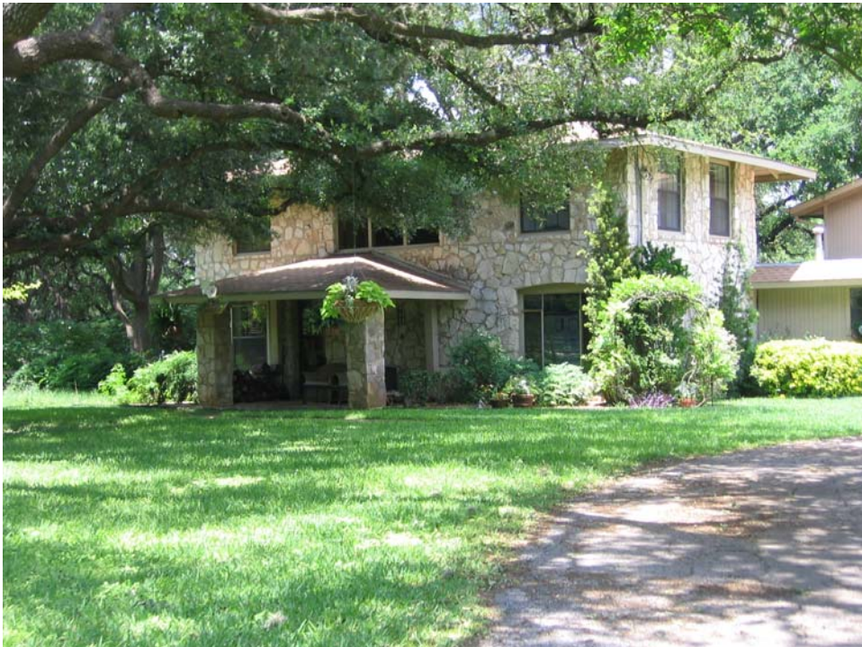
Figure 51: Two Story Lodges
