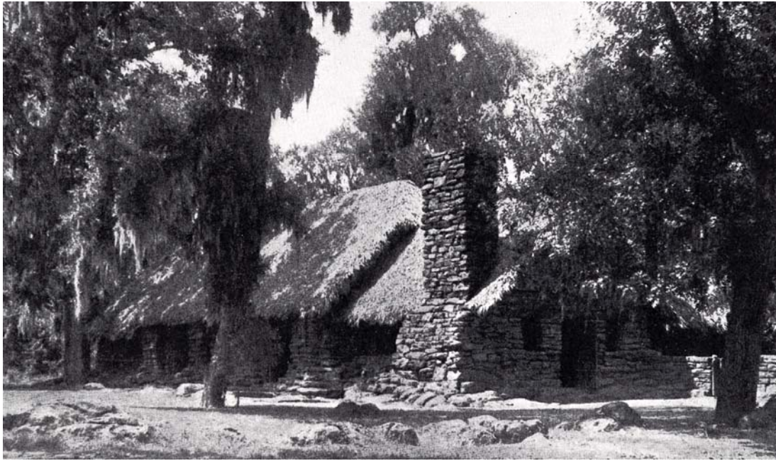
Refectory, Palmetto State Park
